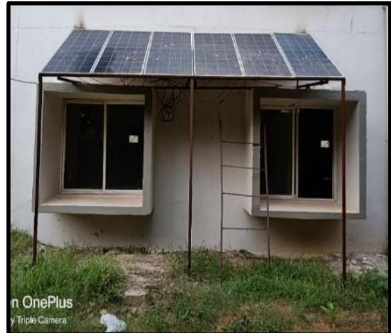
Fig. 20. Installation of solar power plant
