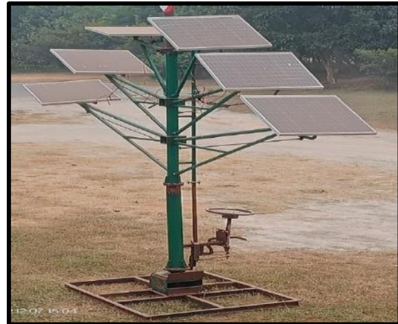
Fig. 17. Installed solar tree
