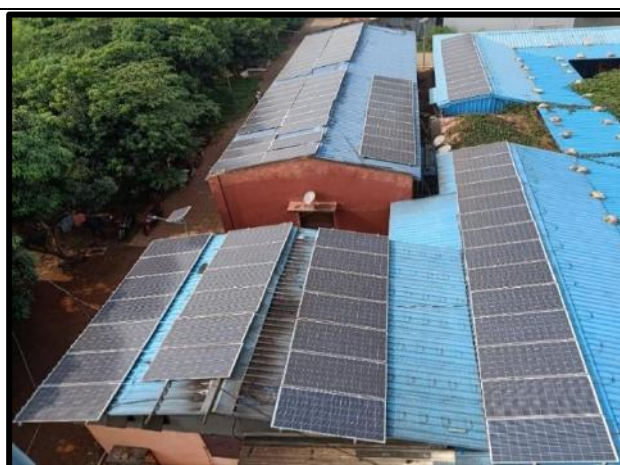
Fig. 21. Installation of solar PV system
