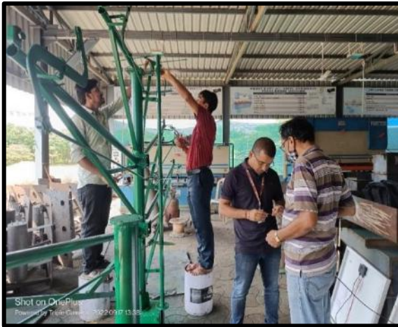
Fig. 16. On-going installation of solar tree
